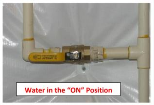
Note: Some City Jurisdictions require a drain on the shut-off line in the basement. This line must also be drained. Place a bucket under the drain and open the drain valve so it is parallel to the line to which it is attached. Leave the drain open and proceed to Step 2.
