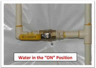
Note: Some City Jurisdictions require a drain on the shut-off line in the basement. Make sure this drain is in the "OFF" position (perpendicular) before turning on the water to the backflow preventor.
